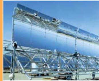
Solar thermal panels
